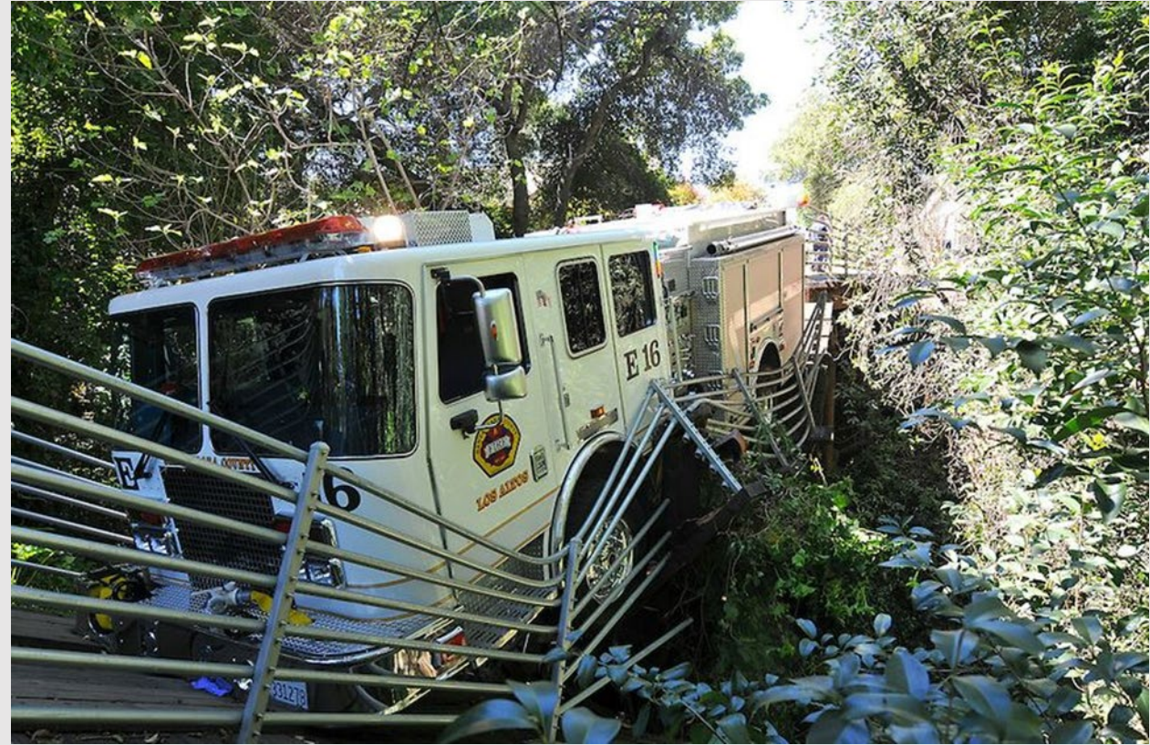
Los Altos, CA, April 2001: A 19-ton emergency vehicle on a bridge that had been rated for 18 tons in 1979.
