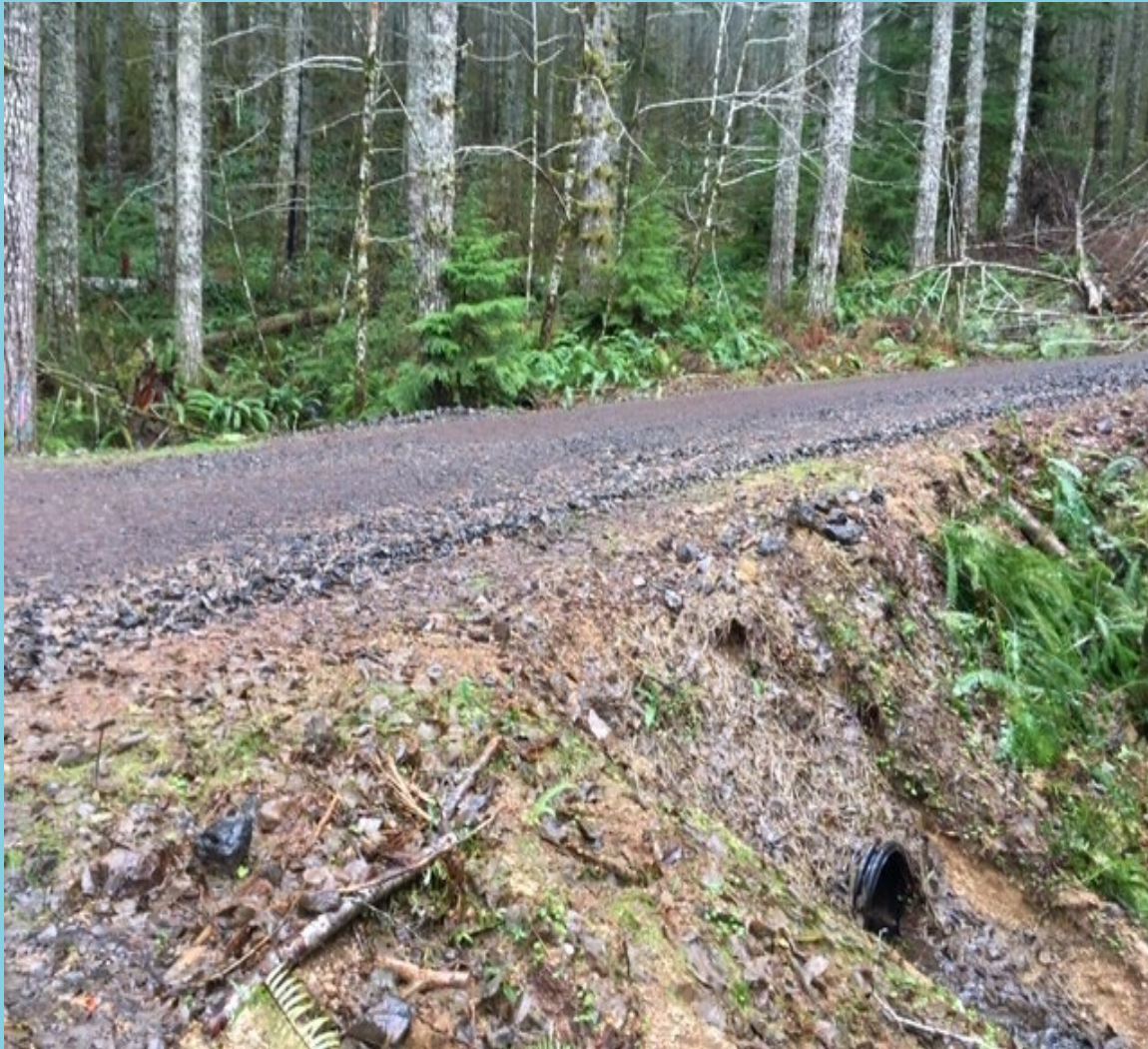
Short pipe (40') limits road width through crossing.
