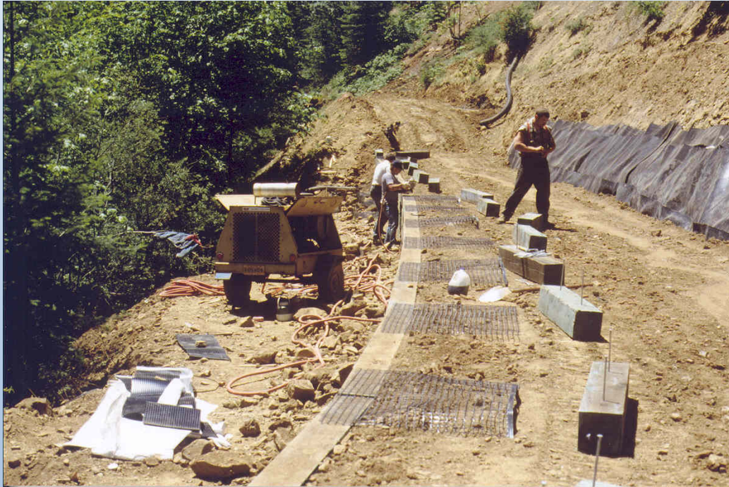
Timber Faced Geogrid Reinforced Wall, Happy Camp R.D. Klamath N.F.
