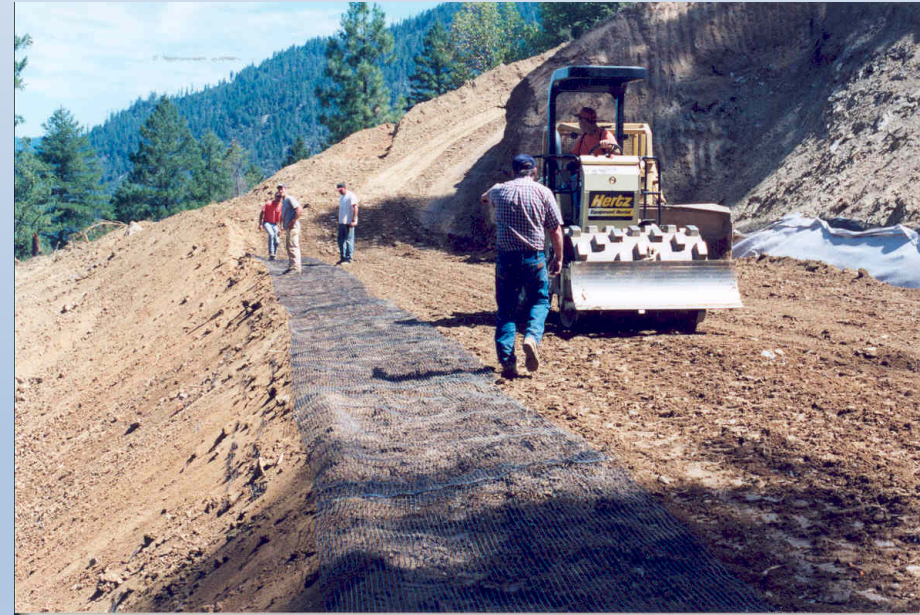
Secondary Geogrid Reinforced Fill Layer. Essential compaction of Soil for Strength
