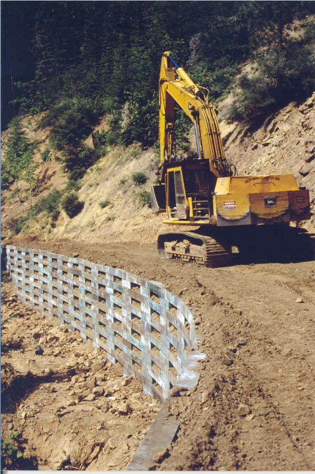
MSE Wall Just after Completion
