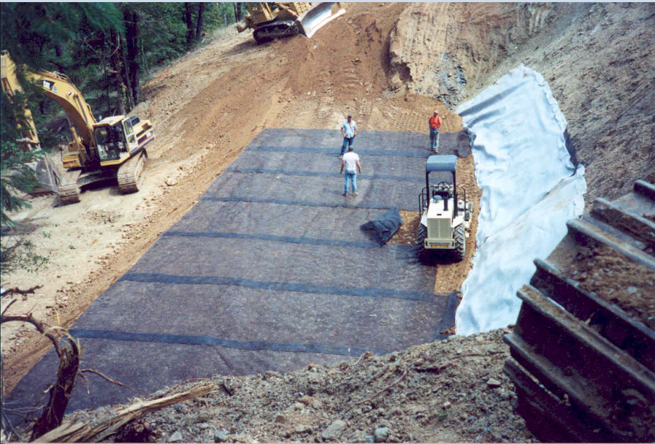
Primary Geogrid Reinforced Fill Layer
