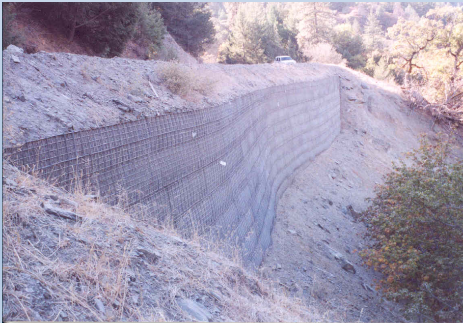
Hilfiker Welded Wire Wall-Mendocino N.F. Region 5
