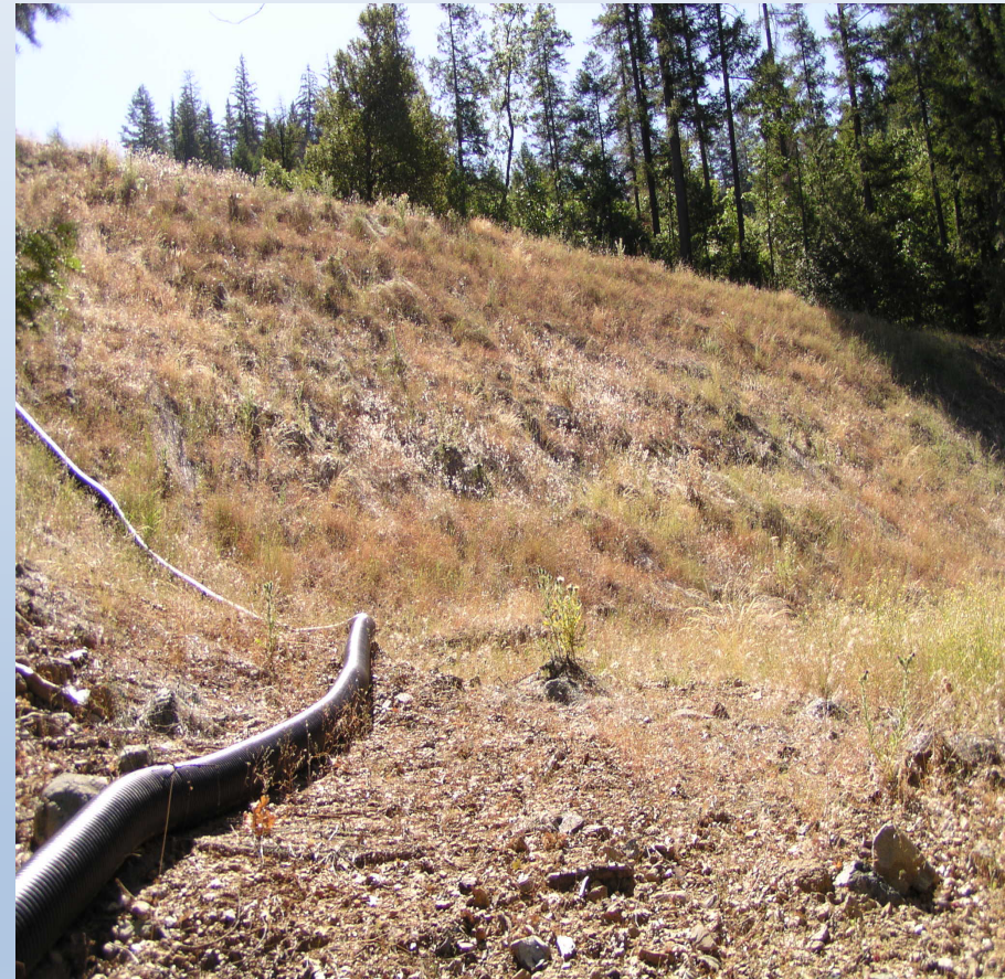
Reinforced fill 2 years after completion.
