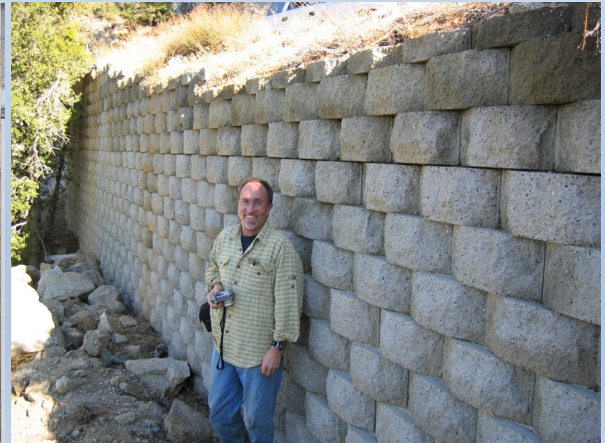
Angeles N.F. Region 5 Geogrid Reinforced Modular Block Wall
