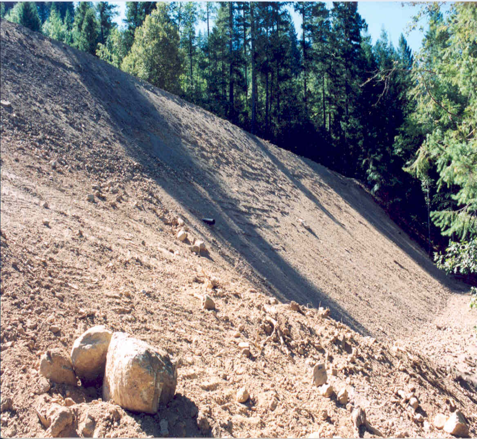
Completed reinforced fill before erosion control mat placed on slope
