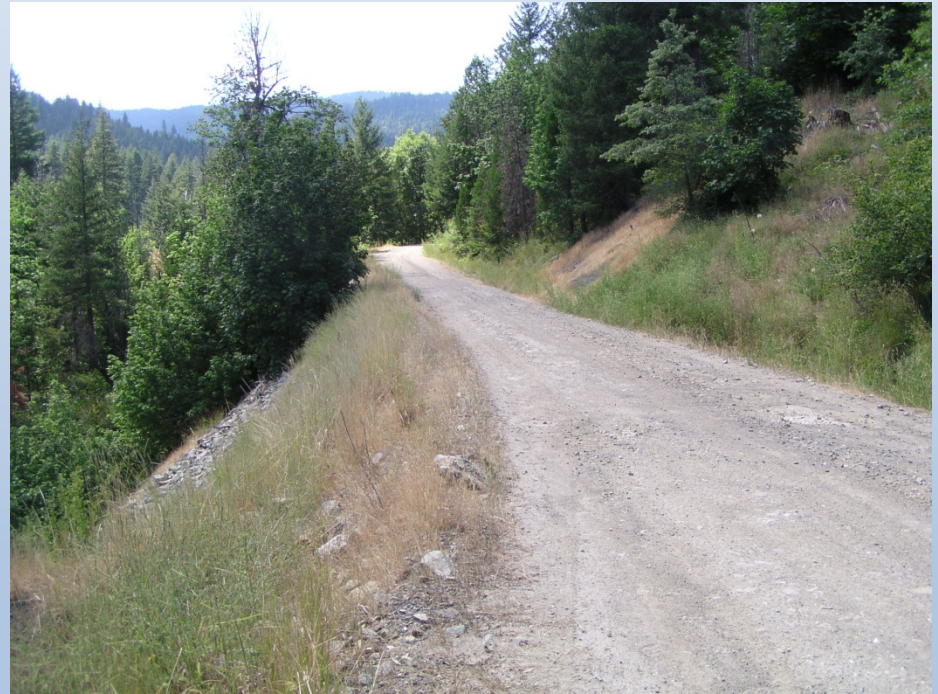
Reinforced Fill 3 years after Construction
