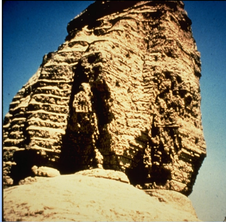
3000 B.C. - Mesopotamia “Reeds” placed in horizontal layers used to reinforce soil
