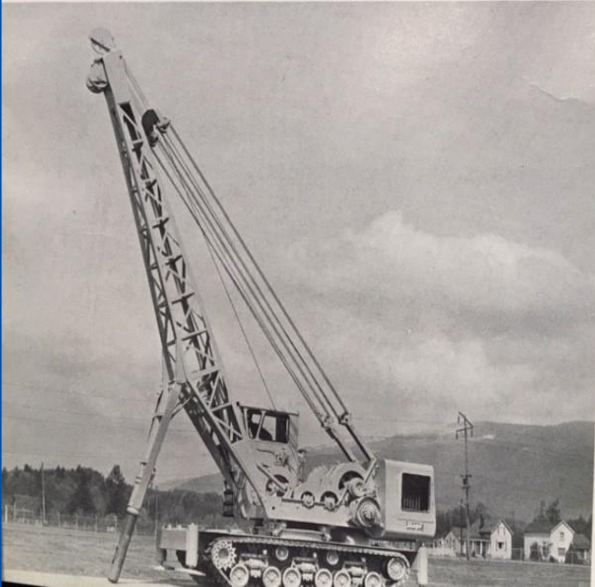
First of the grapple yarders. Skagit GT-5 with Jillpoke, April, 1966.
