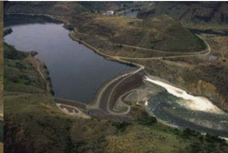
Oxbow Dam (175 ft.)
