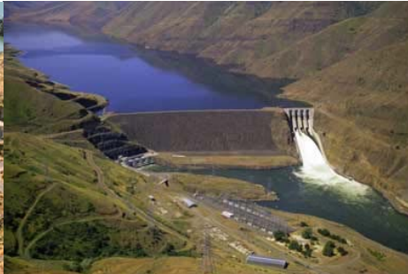
Brownlee Dam (420 ft.)
