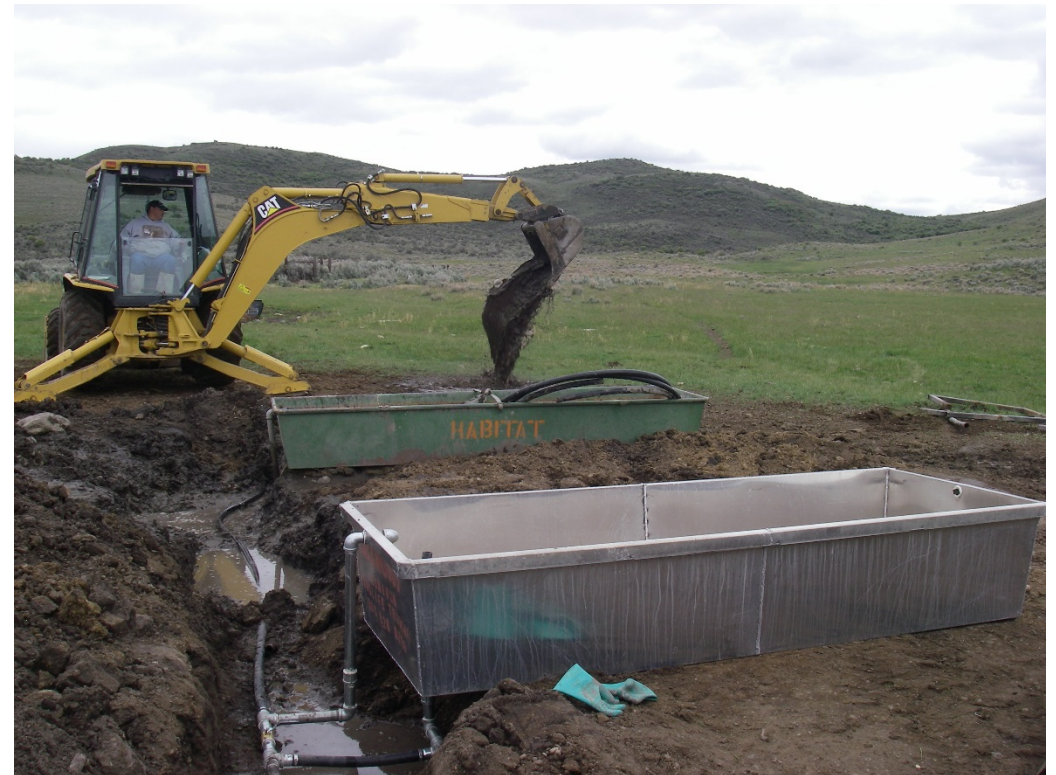
Put in new aluminum Trough at Cold Springs
