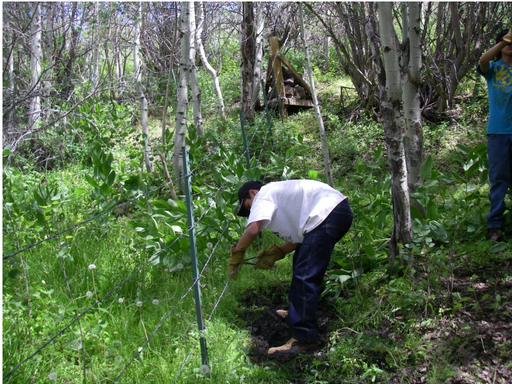
Klein Kelly Summer Youth Worker Doing repairs on fence
