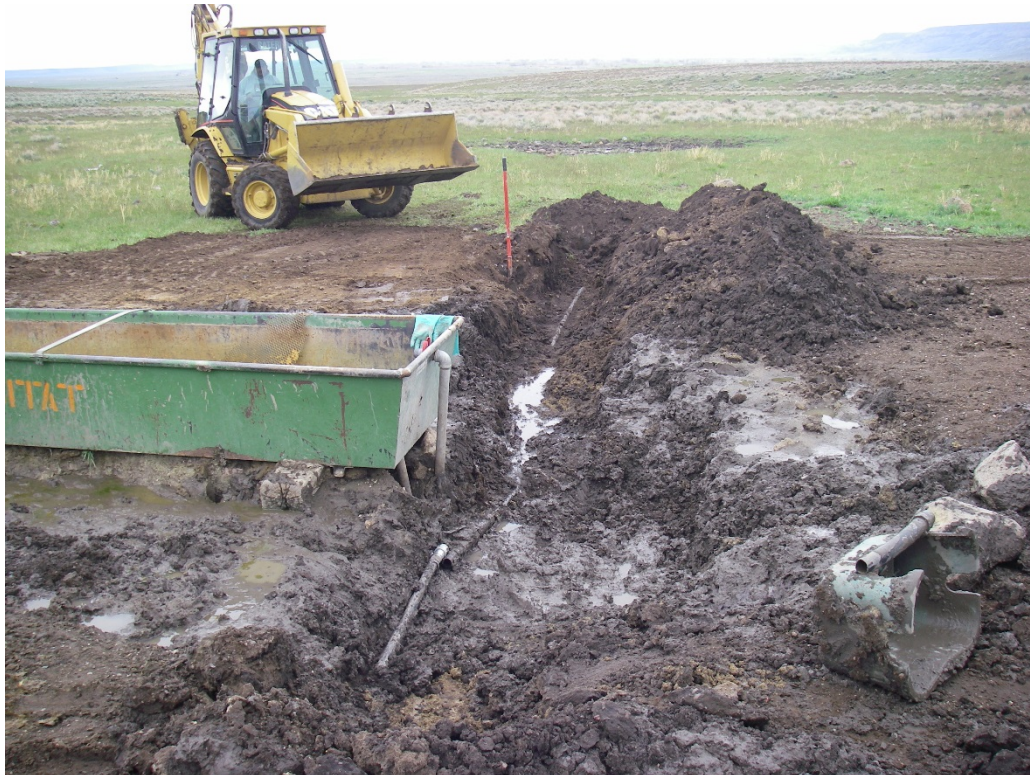
Replacing trough at Cold Springs
