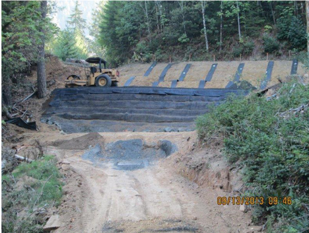
Reinforced Soil Slope near Agness, Oregon
