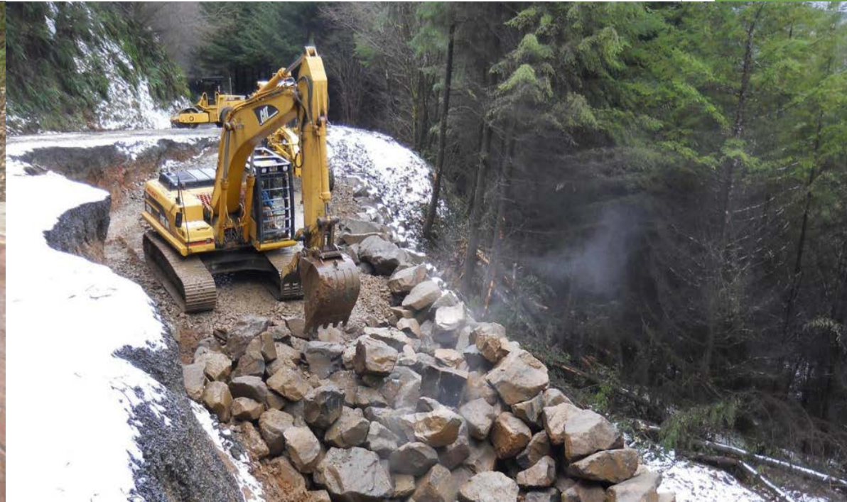
Slide Repair using Boulders and Large Rock
