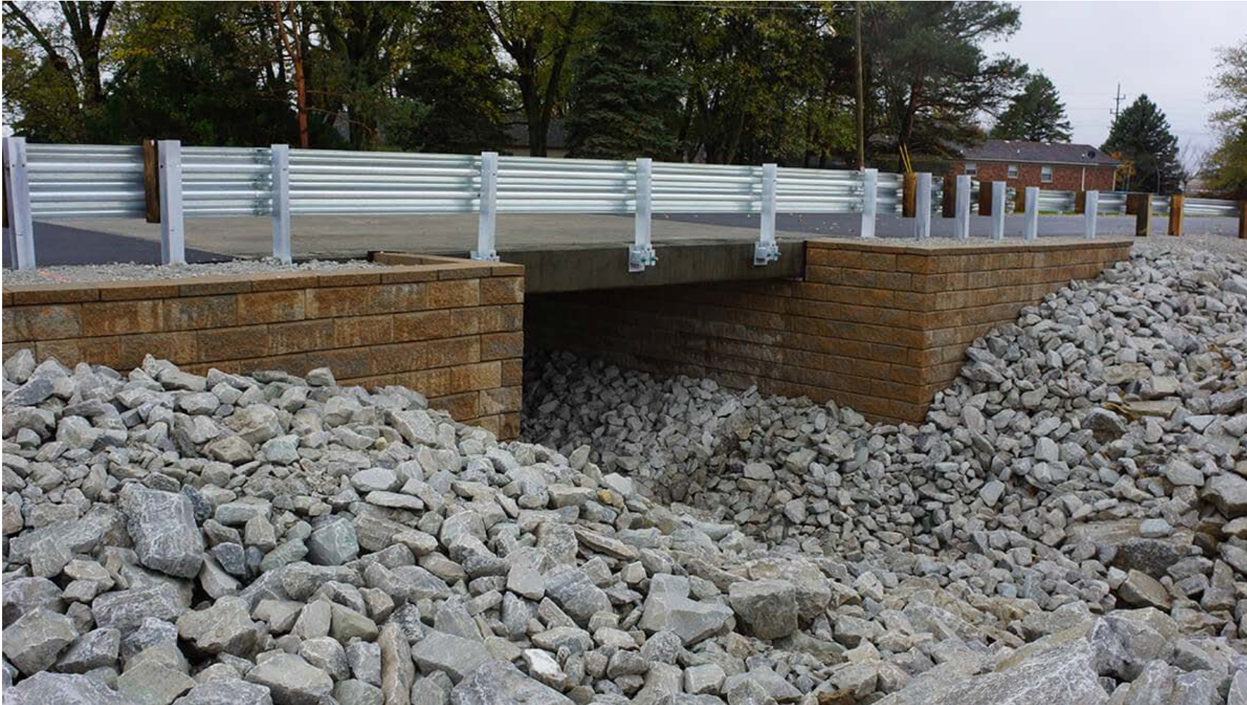
GRS-IBS Bridge Abutments
