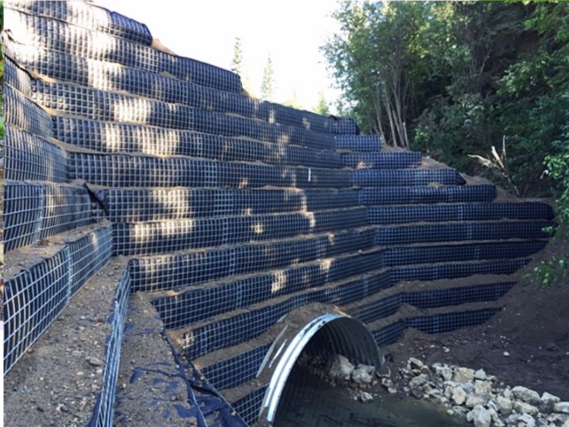
Fish Passage using Corrugate Metal Pipe and GRS
