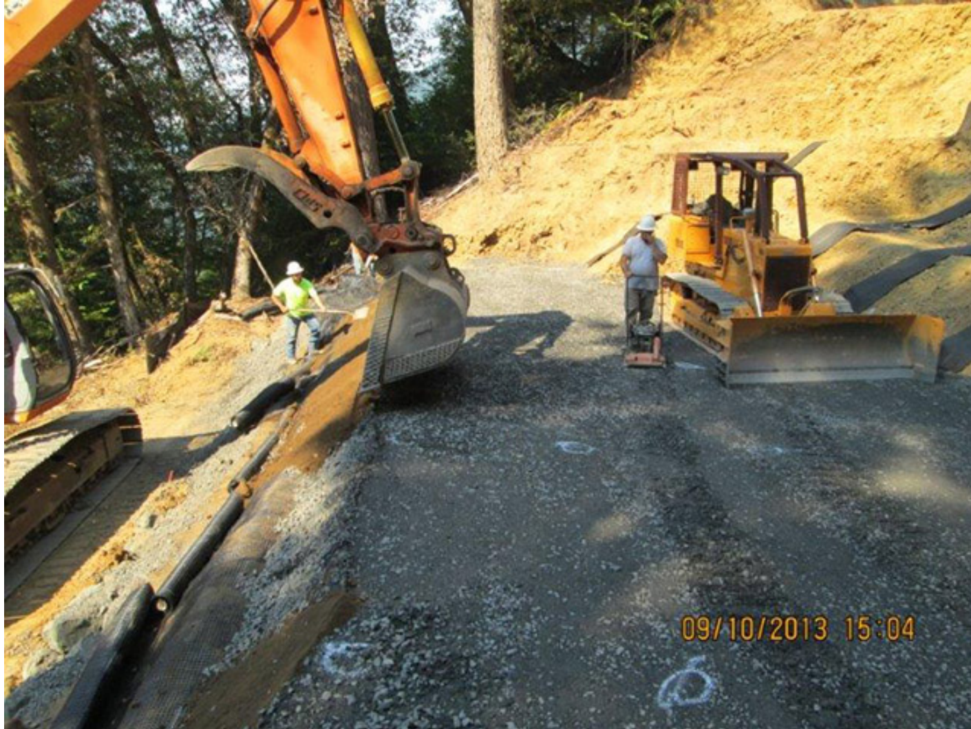
Reinforced Soil Slope near Agness, Oregon
