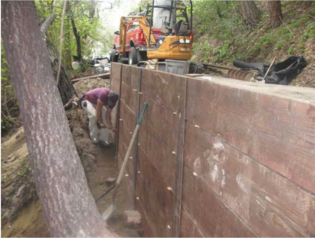
Slide Repair using H-Piles and Timber
