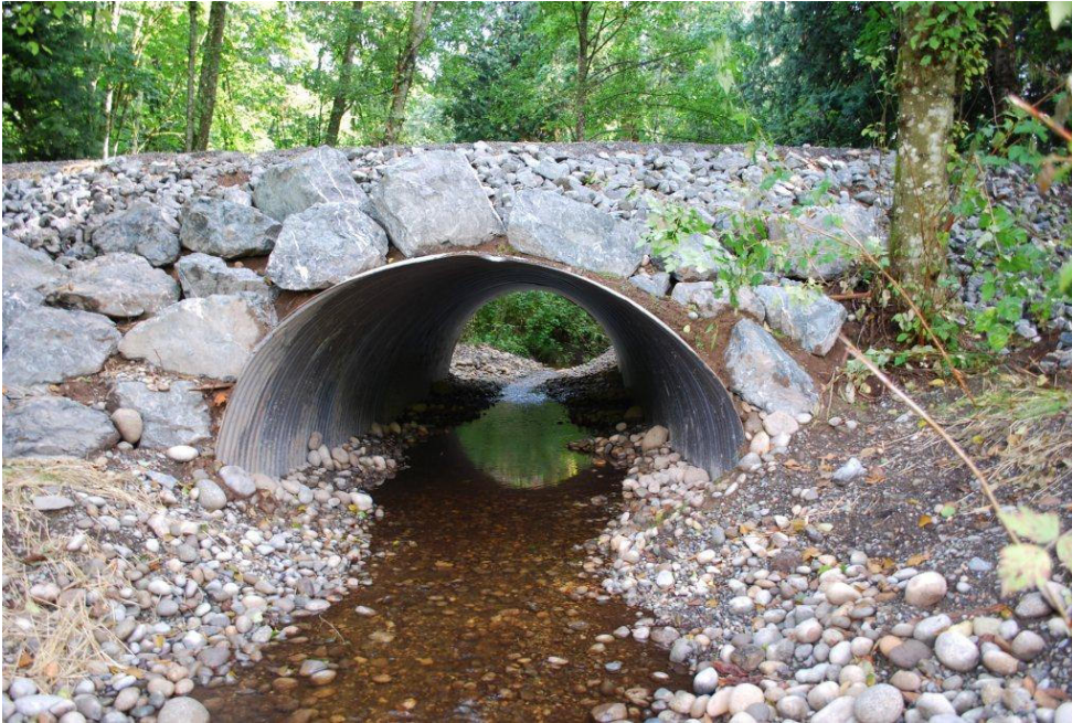
Fish Passage using Corrugated Metal Pipe
